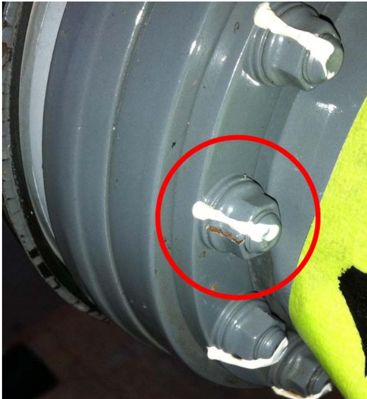
Figure 1 - Example of a failed nut (Courtesy ATSB)
